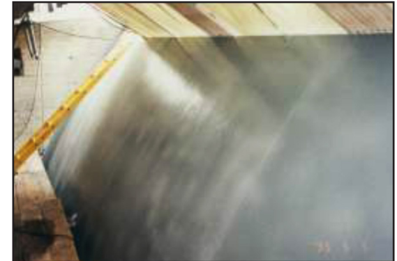
Gate top coated with 2 coats of ARC S2
