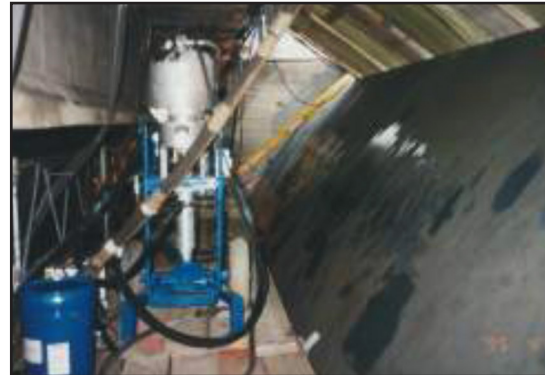
Pitting repaired using ARC 858
